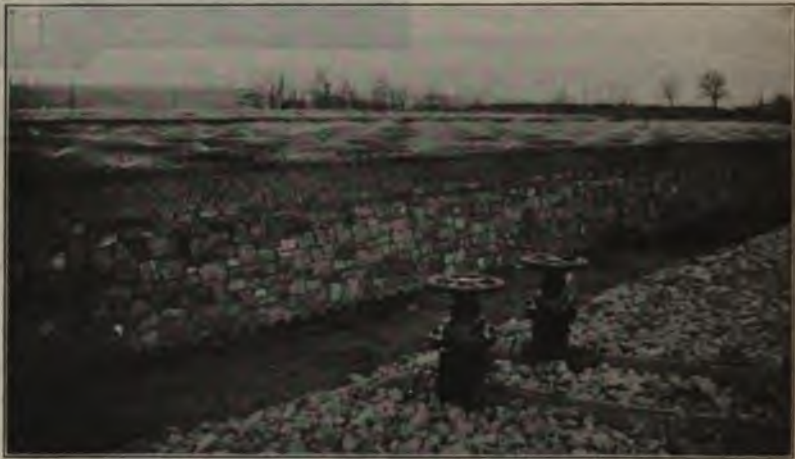
FIG. 129.—TRICKLING FILTER AT BIRMINGHAM, ENGLAND.
