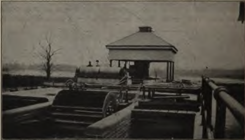
FIG. 126.—INCLINED SCREEN OPERATED BY WATER WHEEL, BIRMINGHAM, ENGLAND.
