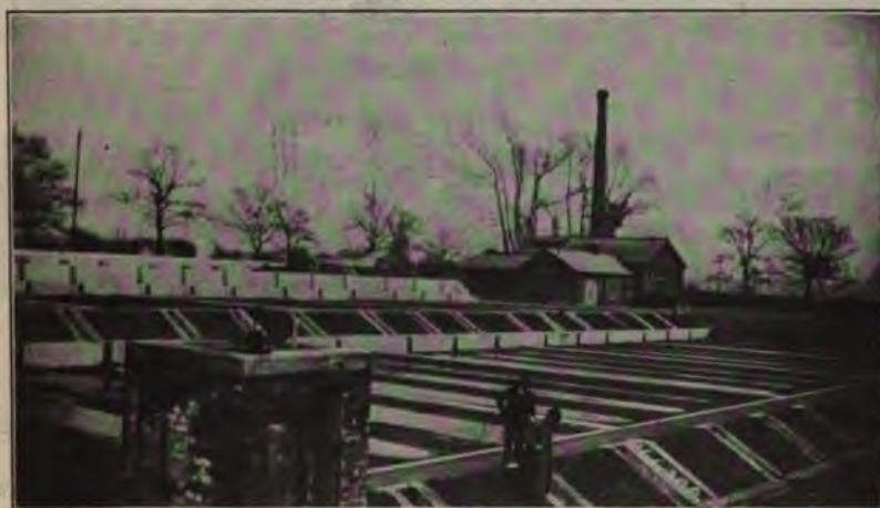
FIG. 124.—TRIPLE CONTACT BEDS AT HAMPTON, ENGLAND.
