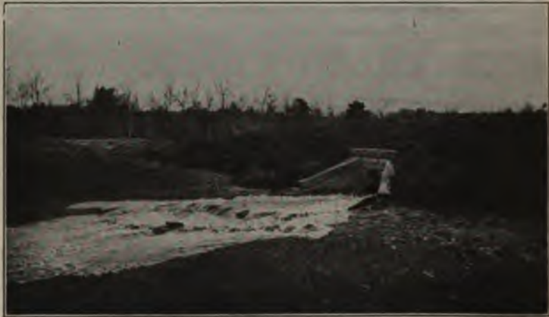
FIG. 133.—DISCHARGE OF SEWAGE UPON A FILTER BED AT BROCKTON, MASS.
