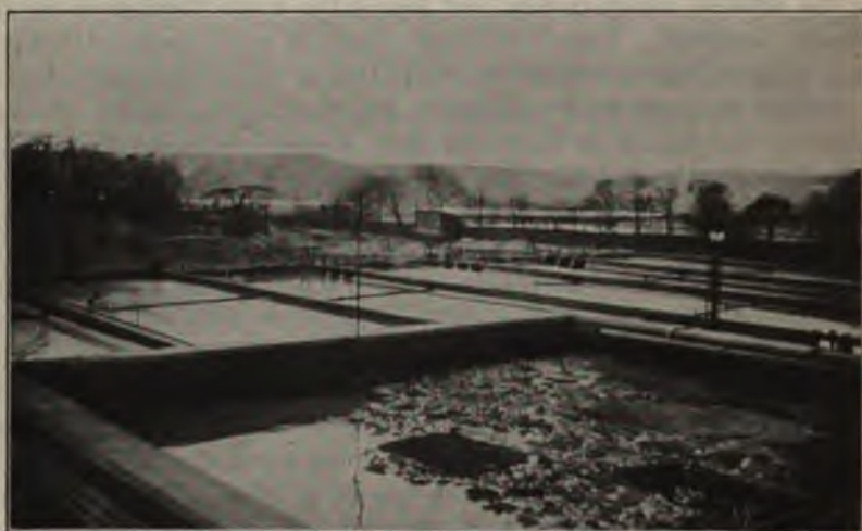
FIG. 130.—SEPTIC TANK AND CHEMICAL PRECIPITATION TANKS AT ROCHEDALE, ENGLAND.
